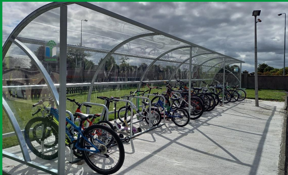
Figure 49 - Cycle parking provided by SRTS was installed in July 2022
