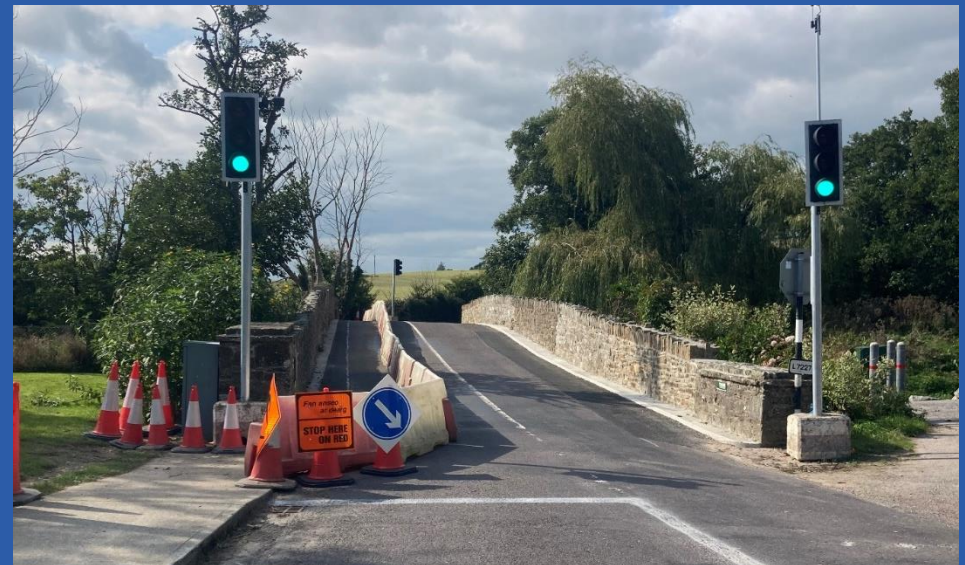
Figure 39 - The shuttle system trial on Aghafantaun Bridge
