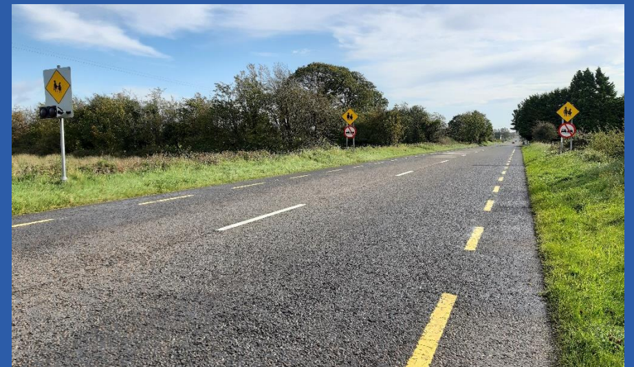
Figure 22 – Existing road composition at the front of school
