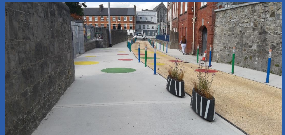
Figure 47 - Roden St. on completion of the works
